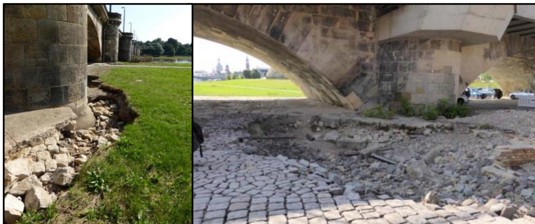
Figure 17. Damage to the front (left) and back (right) side of a bridge basement next to the 2013 flood
