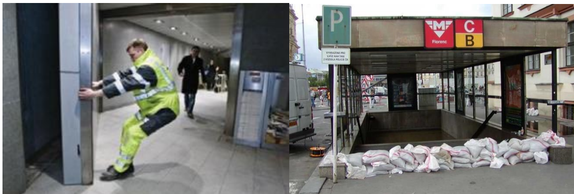
Figure 18. Flooding gates (design) and sand bags (response) to prevent flooding underground stations
